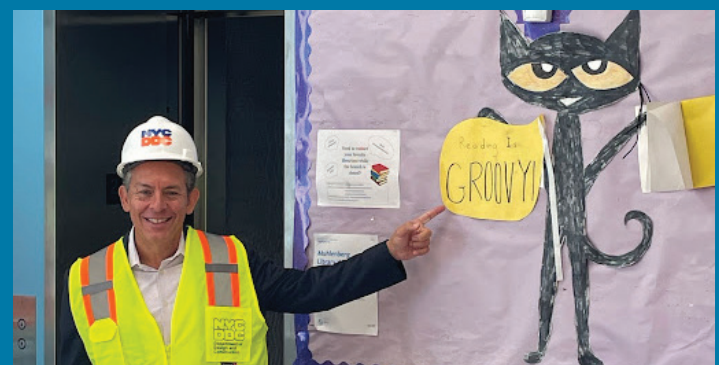
Surveying construction at Muhlenberg Library in Chelsea which is slated to reopen next year after HVAC improvements, elevator repairs, sidewalk improvements and a new fire alarm system.
