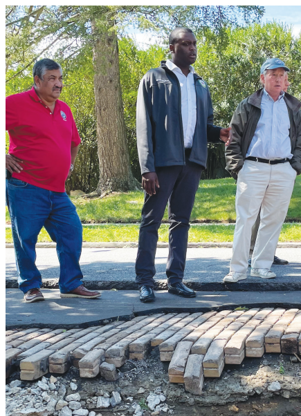
Port Chester Mayor Luis Marino, Congressman Mondaire Jones and Assemblyman Otis surveying road damage on Glen Avenue from the hurricane.
