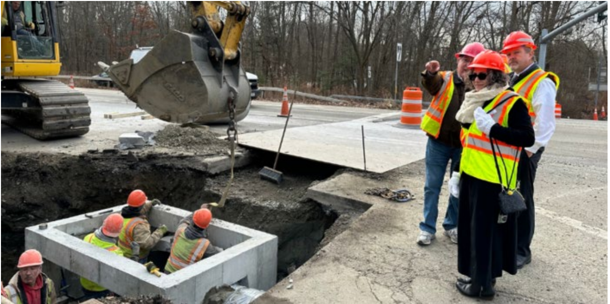
Touring the culvert project at the intersection of Routes 9A and 134.
